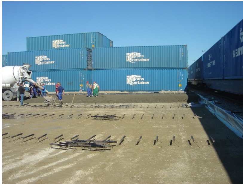
Figure 7. The arrangement of dowels during concreting
