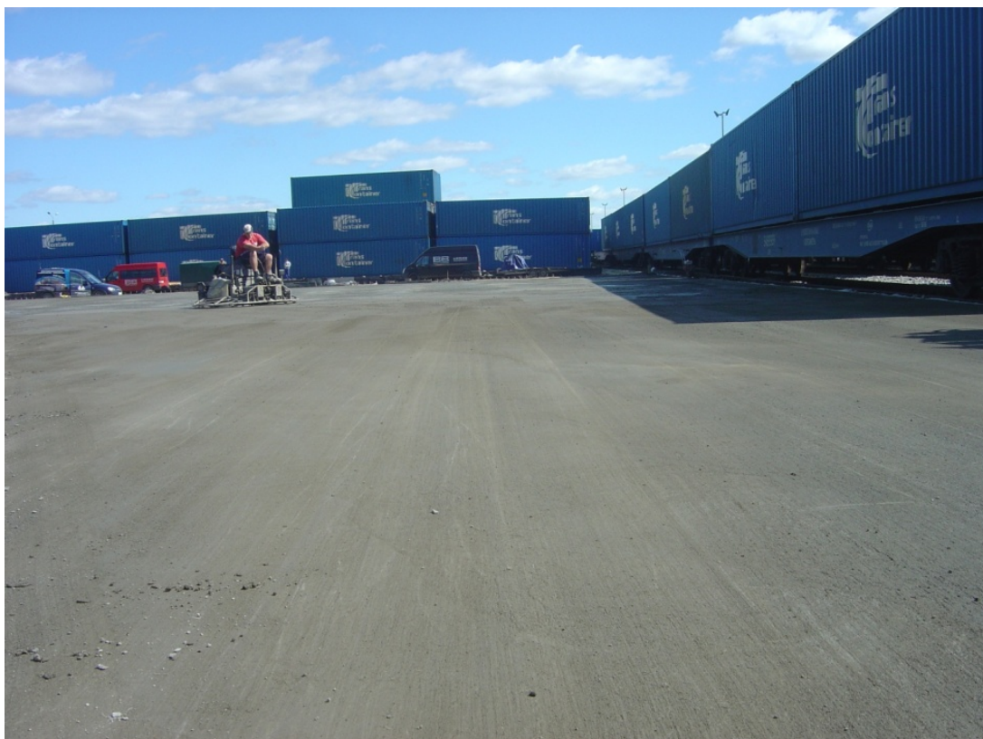
Figure 8. Floating and texturing of concrete pavements
