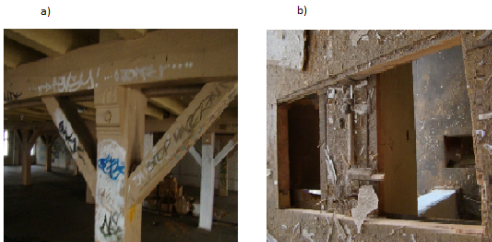
Figure 8. Building planned for modernization ceiling above the first floor: a) fragment of the wooden frame, b) structure of the ceiling
