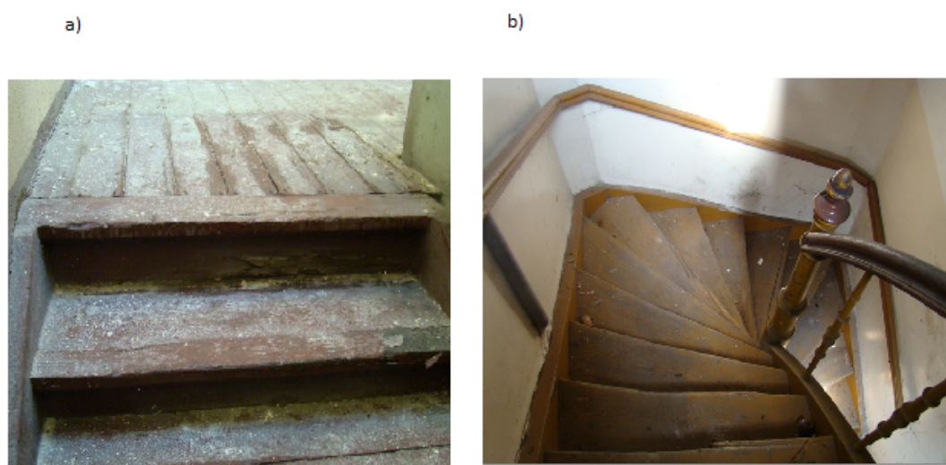
Figure 11. Building planned for modernization - damage to the runs of staircases: a) main and b) side
