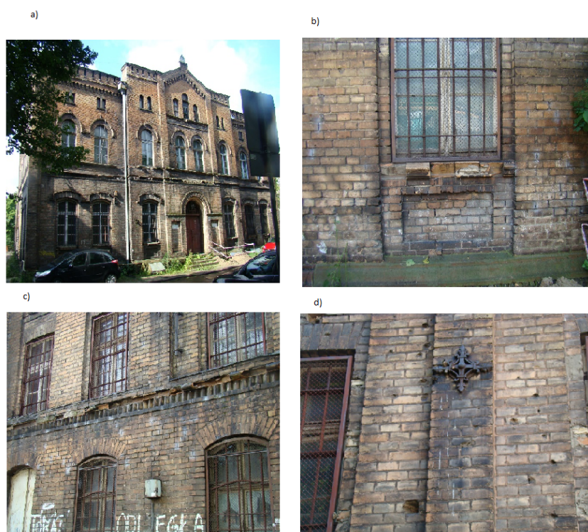
Figure 3. Building planned for modernization - elevations: north-east: a) view, north-west: damage to: b) the sill zone, c) brick basement window lintels (arches), d) front anchoring retaining plate
