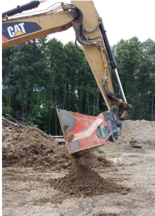
Figure 1. Crushing cohesive soil with a recycler
