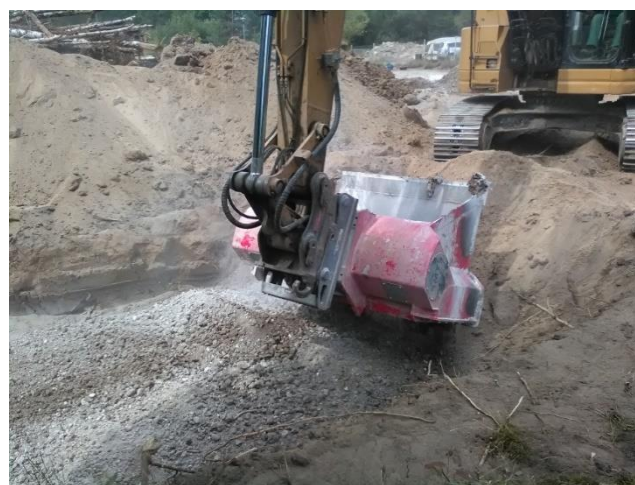
Figure 5. Filling a layer of soil mixed with lime into a excavation
