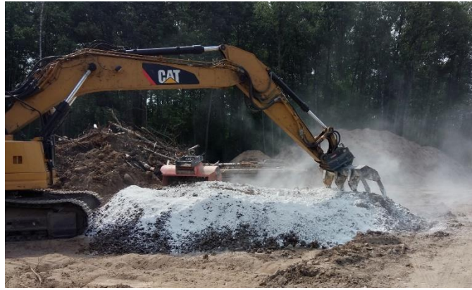
Figure 3. Mixing soil with quicklime using a blade rake
